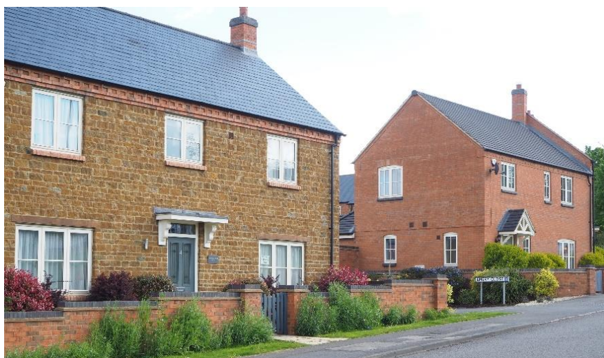
Emery Row - recently completed housing development
